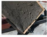
HVAC filters should be replaced or cleaned. Air return plenums, A/C coils and blowers should be wipe-tested and cleaned if necessary. Ventilation systems operating during a fire event may be impacted throughout, with deposits generally greater on the return side. Sampling of supply
