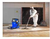
Removal of loose combustion particles is a universal first step. Freshly settled ash and char are lightly bonded and preexisting dust insulates the surface. Removal of particles at this stage simplifies later procedures and may prove
